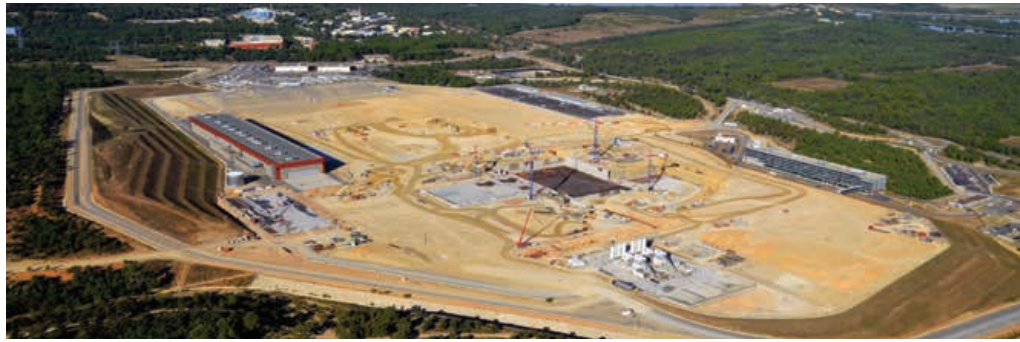
ITER construction, Cadarache
