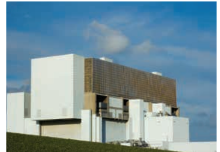
Advanced Gas Reactor - Torness
